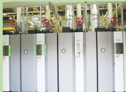
Small once-through boiler installed at the Higashi Ogaki Plant
