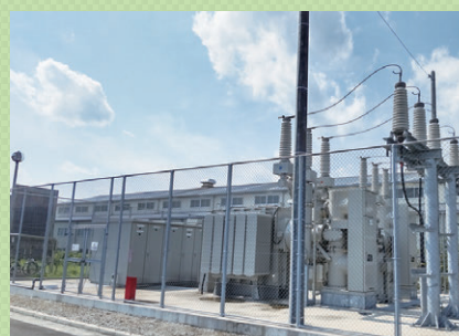
Special high-voltage power receiving equipment at Higashi Ogaki Plant
