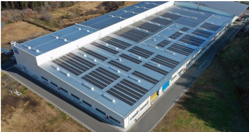
Kurihara Plant with solar panels installed
