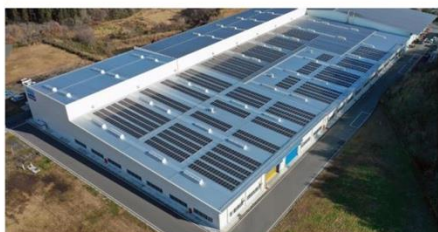
Kurihara Plant with solar panels installed
