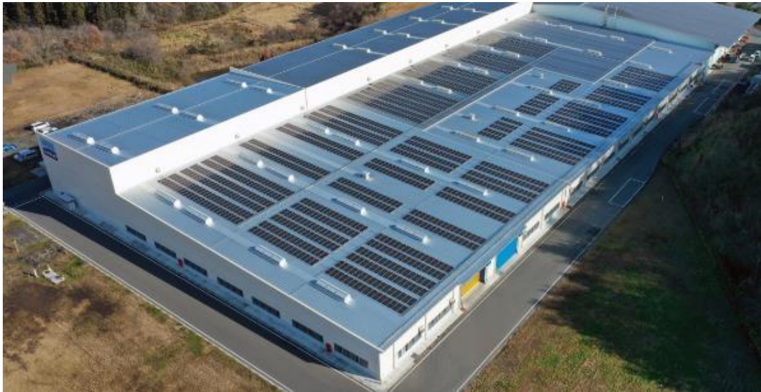
Solar Plants at Kurihara Plant
