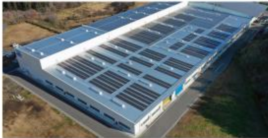
Solar Plants at Kurihara Plant
